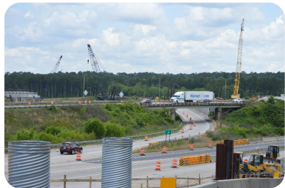
I-16/I-75 Interchange Improvement Project
